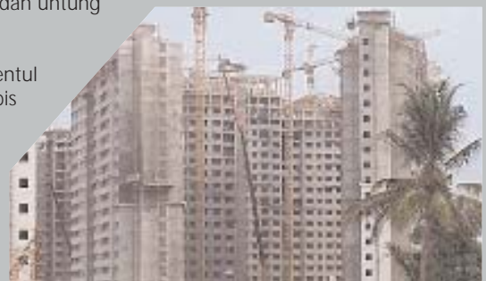
Sri Rampai project in progress
